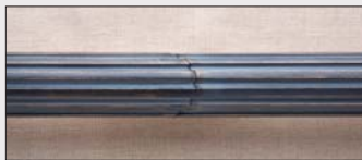
standard 45° splice (for poles and fascia)
